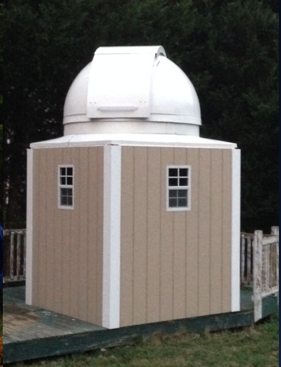
Final construction of Technical Innovations Dome on top of 7x7-foot observatory building
